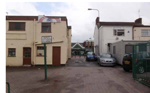
Poor quality pedestrian linkage/route
